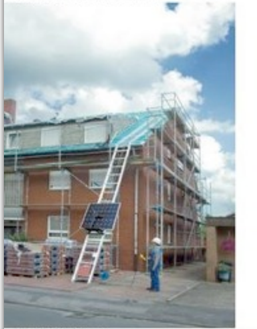
Solarlift to roof
