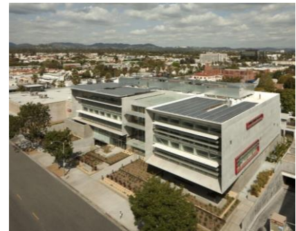
Figure 4. UCLA Health System rooftop solar.
