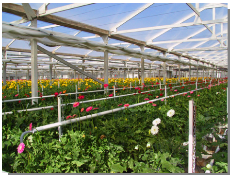
Waste heat from the internal combustion engines is utilized for nutrient processing and heating 12 acres of greenhouses.
