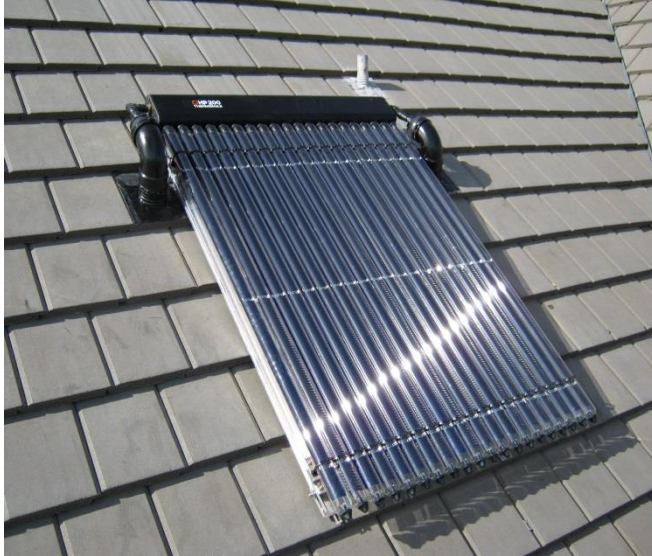
Evacuated Tube Collectors
